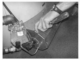
Step 1: Remove burner box cover screws
